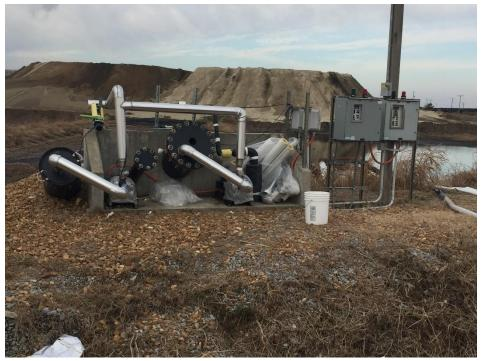
2. Cell 15 leachate collection riser pipes and controls looking west. An additional riser pipe, pump and control panel was installed in 2018.
