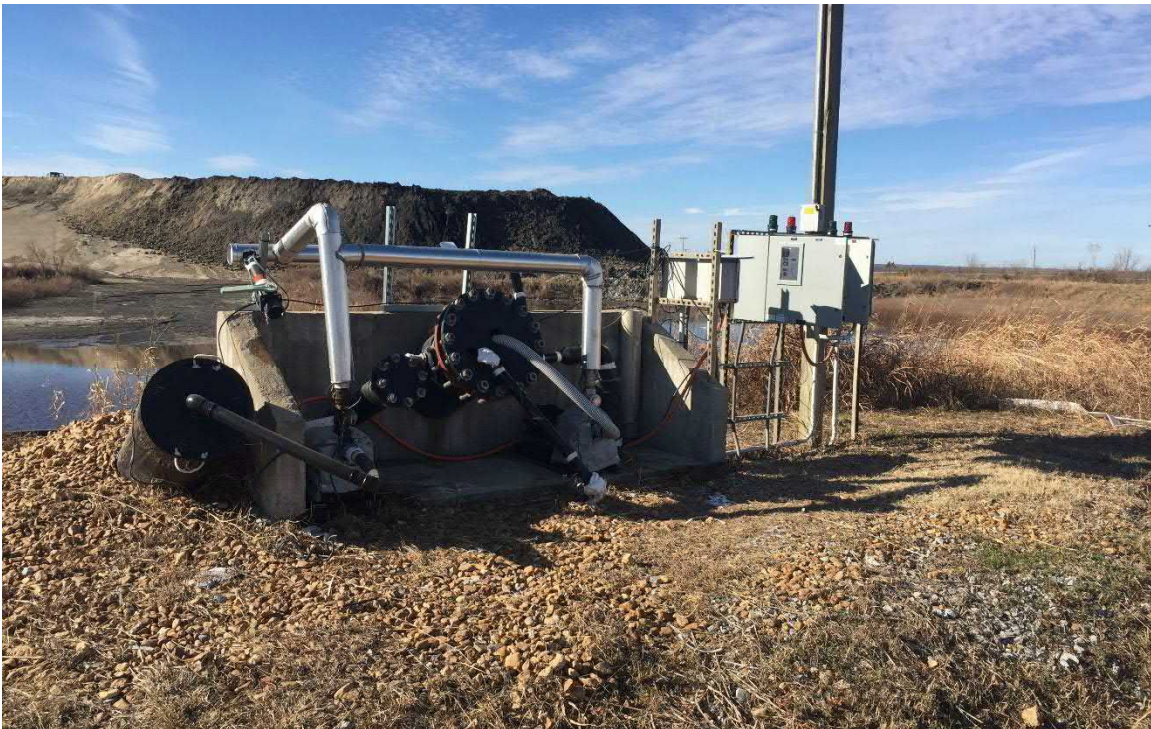
2. Cell 15 leachate collection riser pipes and controls looking west.
