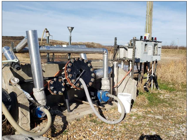
Photo No. 5 Looking northwest at the Cell 15 leachate collection riser headwall and pump control system.
