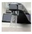
Low flow aerators reduce the amount of water used in older hand washing faucets while reducing the energy needed to heat the water.
