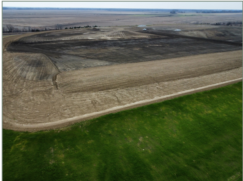
Photo No. 8 Looking northeast at the top deck of active Cells 12, 13, and 14.
