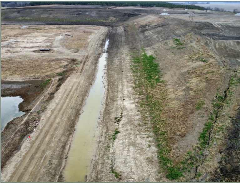
Photo No. 4 Looking northwest at the south slope of active Cell 15.
