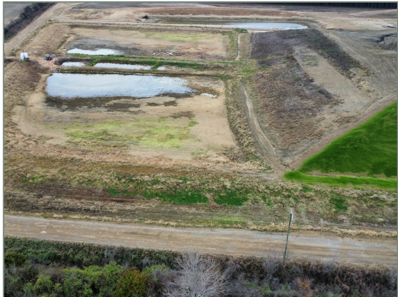
Photo No. 2 Looking southeast at active Cell 15.
