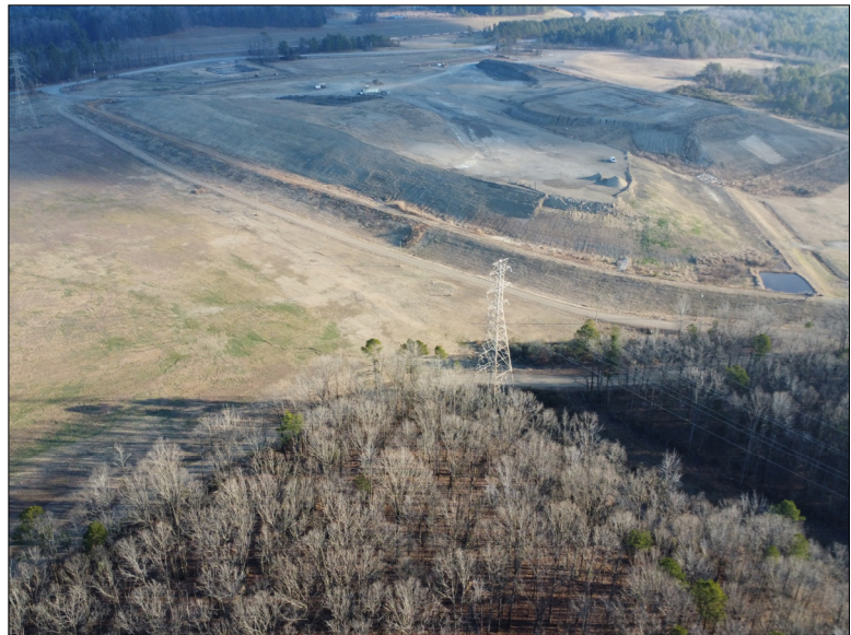
Photo No. 8 Looking northeast at the west side of the Landfill.
