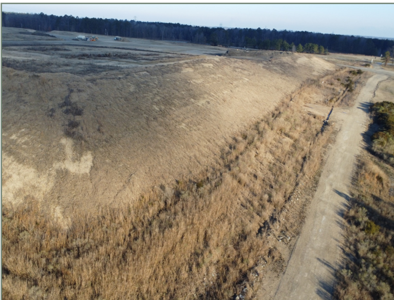
Photo No. 3 Looking north at the east slope of Cell 1 and Cell 2.
