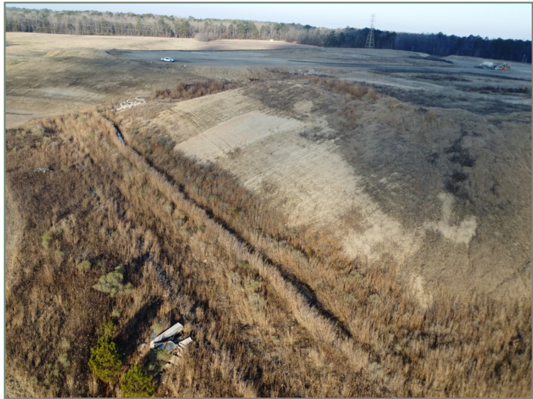
Photo No. 2 Looking northeast at the south slope of active Cell 2.
