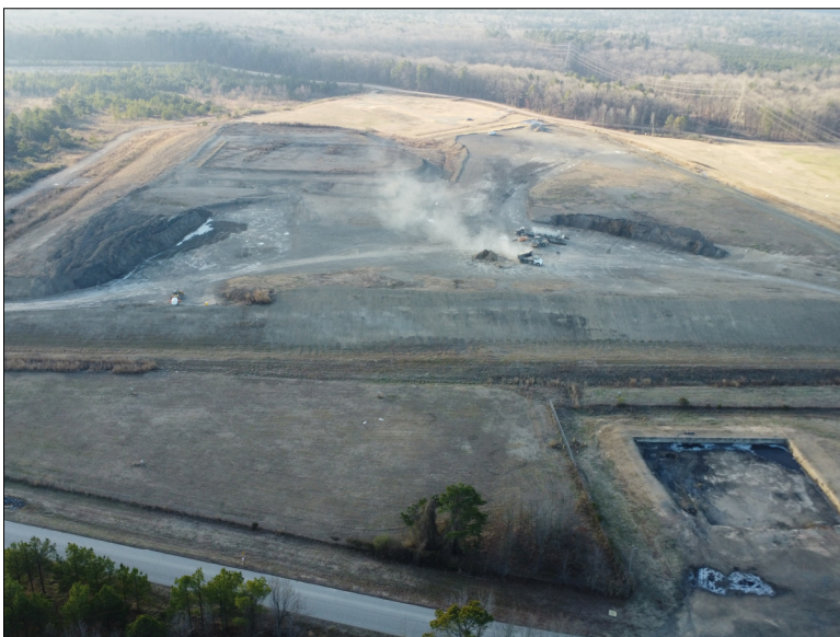
Photo No. 6 Looking south at the active operations of the Landfill.
