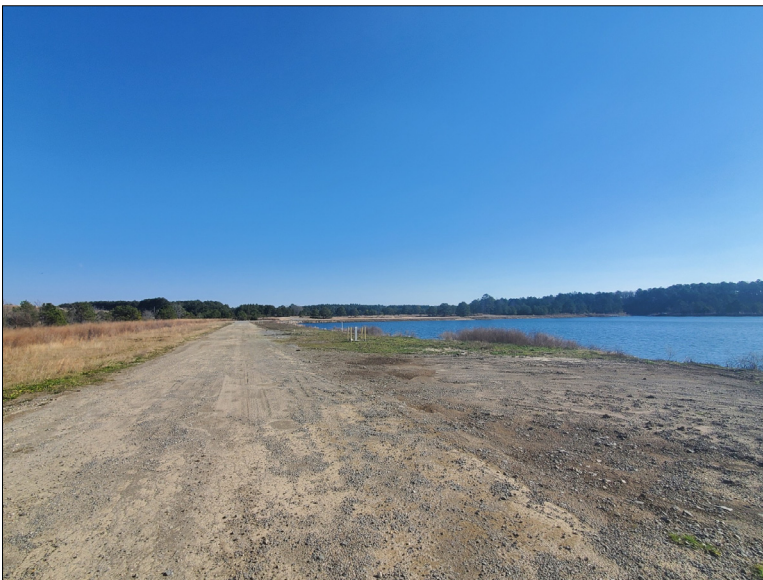
Photo No. 3 Looking east along the north end of the Recycle Pond.
